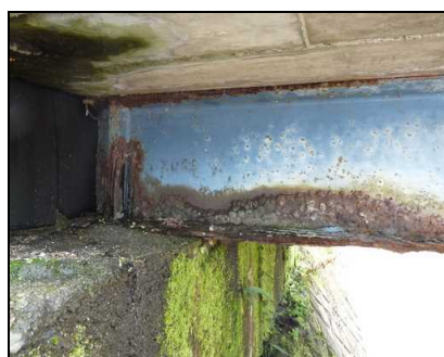
▲鋼橋の損傷
